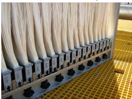
Figure 1: Hollow Fibre Membranes
