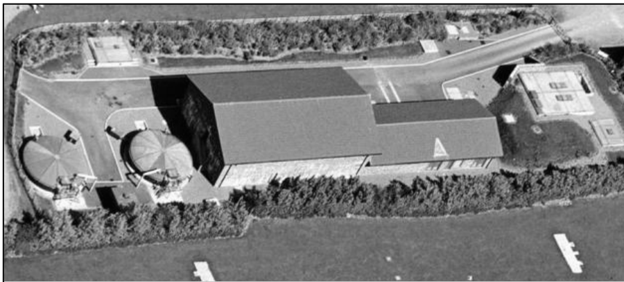
Plate 1: The Porlock MBR wastewater treatment plant in the United Kingdom.
